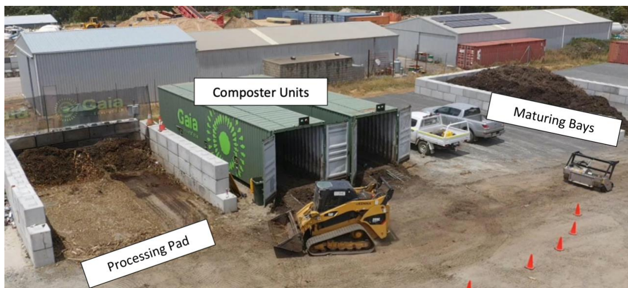
Figure 4-5: Example composting processing set-up
